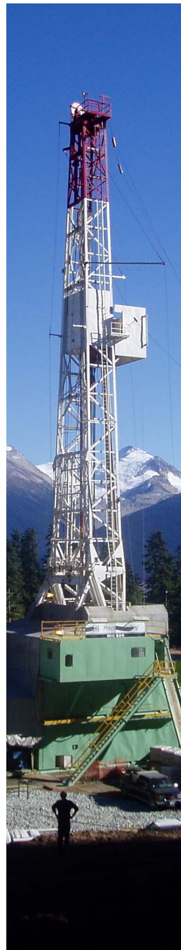
Drilling at South Meager Geothermal Project, B.C. Canada
